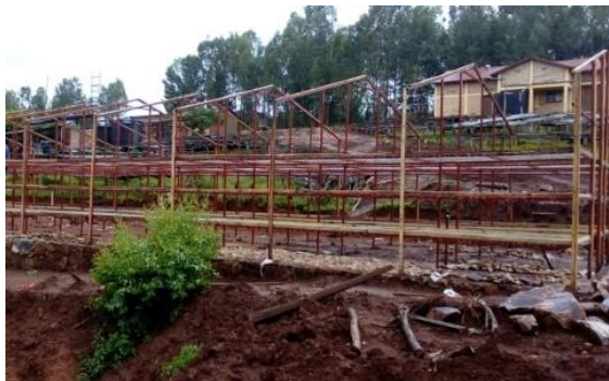
Abahuzamugambi's solar parabolic dryer was set up at their Sovu coffee washing station. A solar parabolic dryer is an improved and advanced greenhouse solar dryer, which is typically used for drying food and agricultural commodities. It contains a parabolic reflector that concentrates sunlight to generate higher temperatures and to accelerate the coffee drying process
